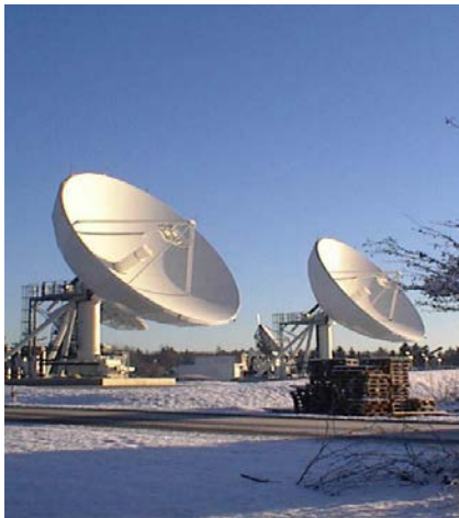
Meteosat antenna Usingen, Germany
